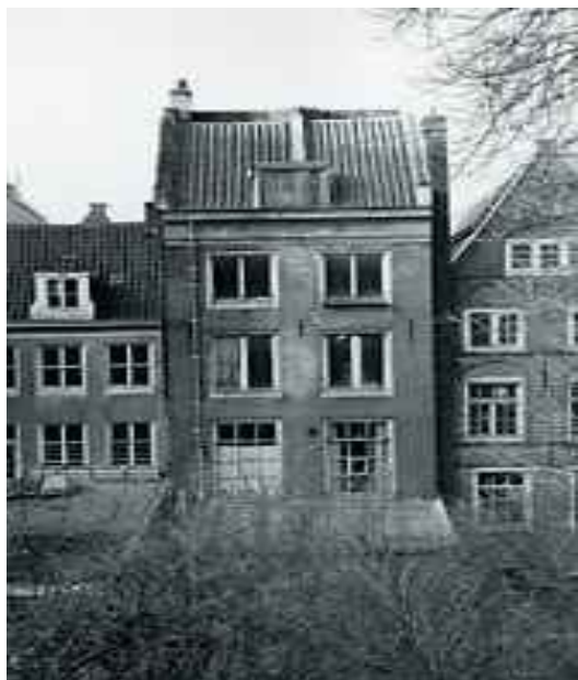
A view of the back exterior of the annex
