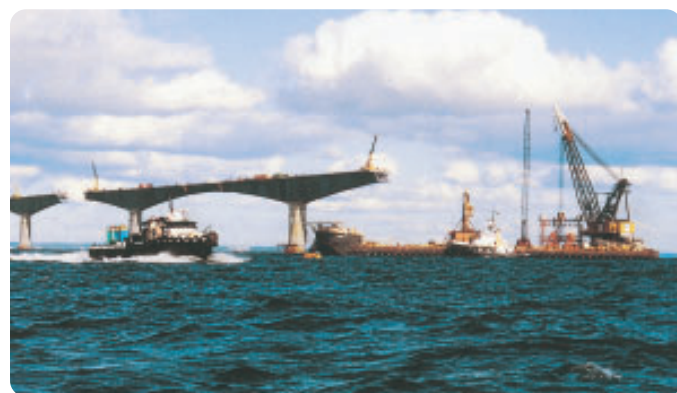
Figure 3 A section of the Confederation Bridge
