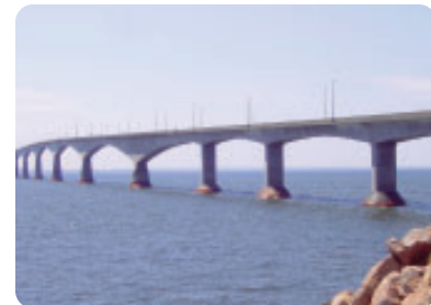
Figure 1 The Confederation Bridge connects Prince Edward Island to New Brunswick.
