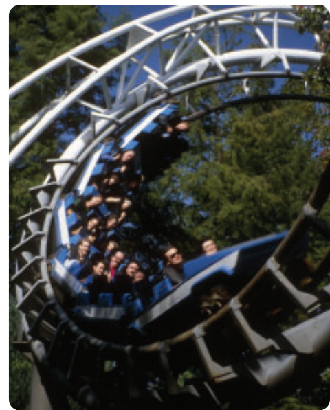
Figure 2 A pneumatic system is used to slow and stop roller coasters.
